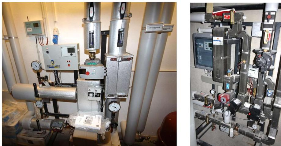
**Fig. 3: District heating transfer stations in two of the studied buildings (Pictures: PHI)**
