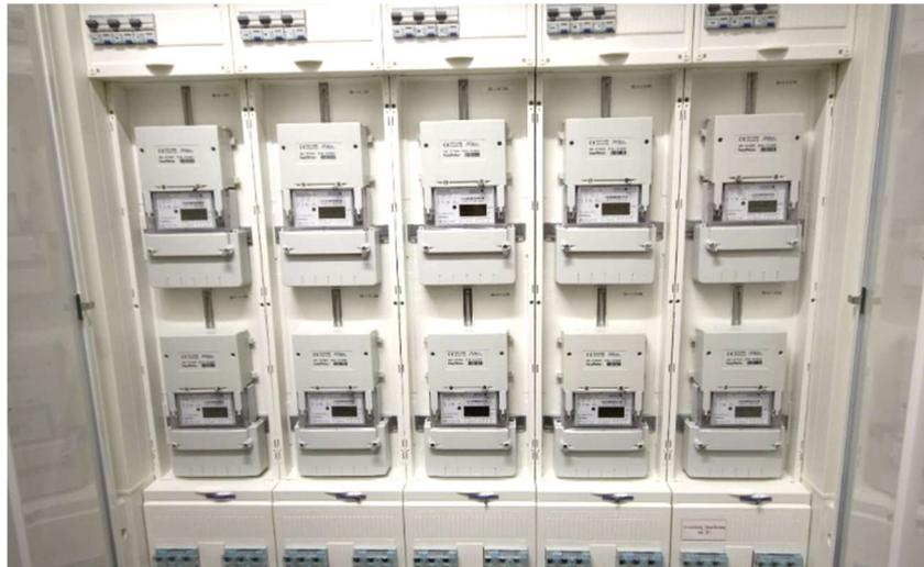
Fig. 20: 10 examples of the ca. 1200 smart meters in one of the investigated buildings (utility room).
