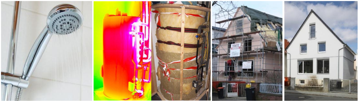
Three examples of changes through which dependence on fossil-based energy can be reduced immediately, over a short time, and in the medium term (from the left): a water-saving shower head, subsequently installed insulation of a hot water tank (with recycled material in this case) and a high-quality deep retrofit of a building. © Passive House Institute
